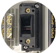
Example of internal 1-pole switch
